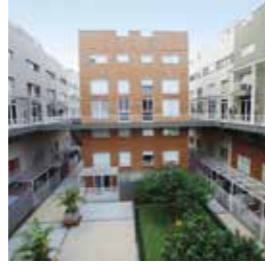
05 | Town Houses Schell Casas en condominio 2007
